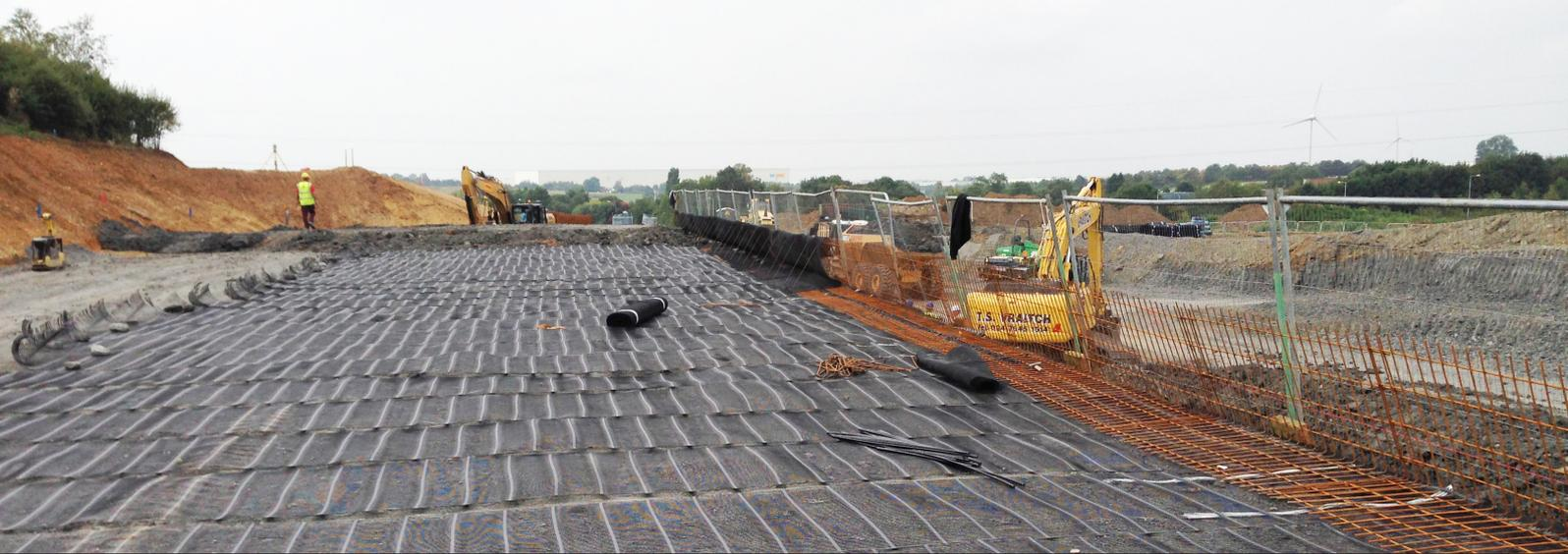
Tensor uniaxial geogrids reinforce the fill used to build the 15.5m high earth bund.
