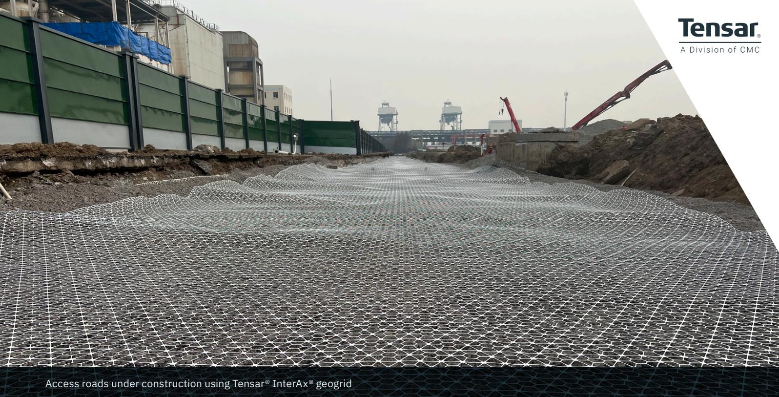
Access roads under construction using Tensor® InterAx® geogrid
